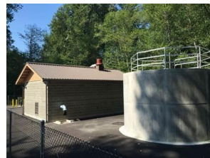
Trail Well Treatment Facility building and Backwash Recycle Reservoir
